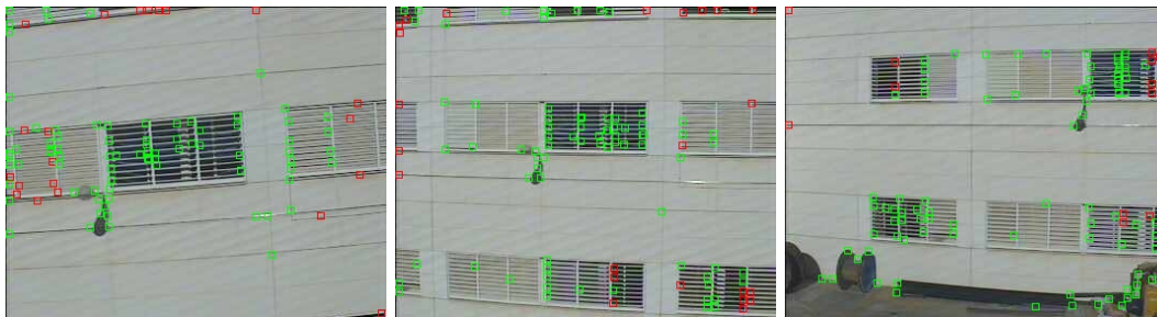
Figure 7.12: Frames 26, 96 and 140 of a building inspection sequence 1.
