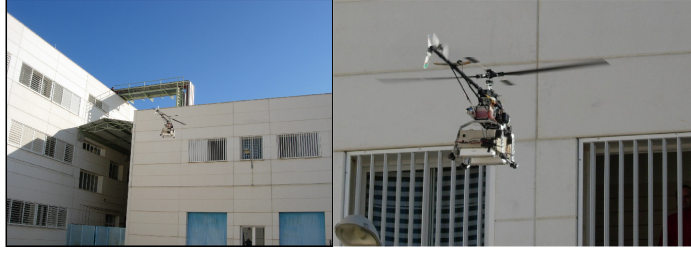
Figure 7.3: The Hero helicopter in building inspection operation.
